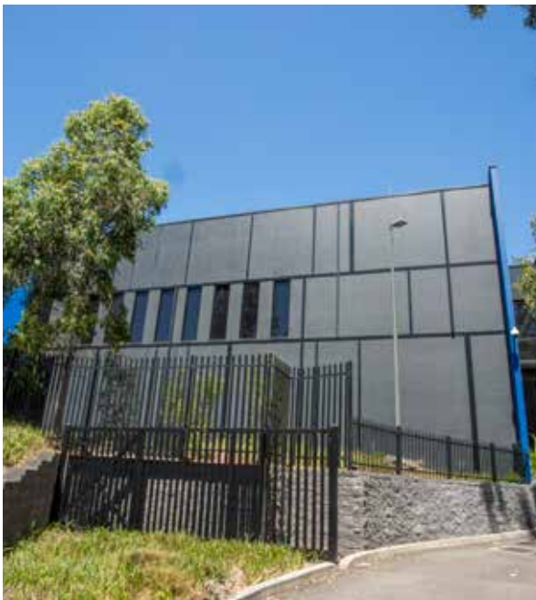
● BKH Contractors Talavera Road, North Ryde
