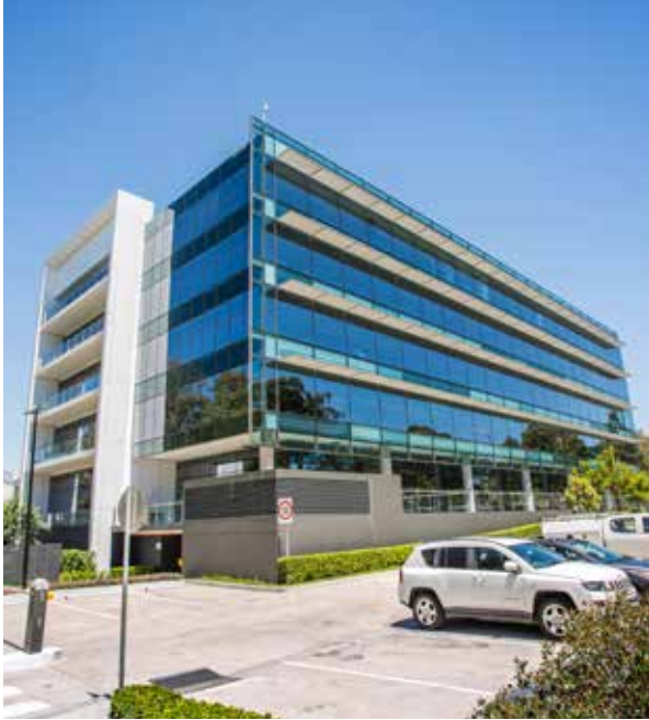
● Presmist Formwork Contractors Talavera Road, North Ryde
